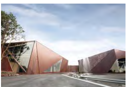
„Privy Council“ Office Building, Beijing, CN China National Academy of Painting, Beijing Beijing Xiangrun, Beijing TECU® Classic
