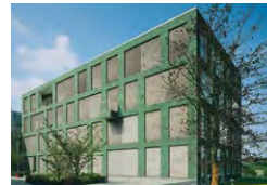
InnovationsCampus, Wolfsburg AG, Wolfsburg, D O.M. Architects BDA, Braunschweig Bisping GmbH & Co., Münster TECU® Patina_mesh
